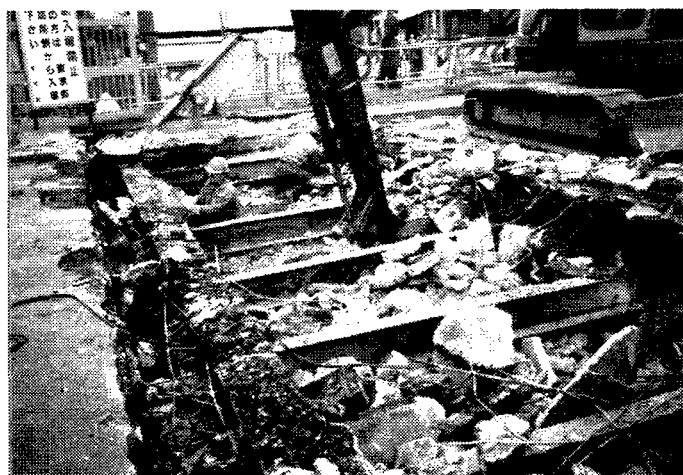
[写真-4.19：床版の撤去]
