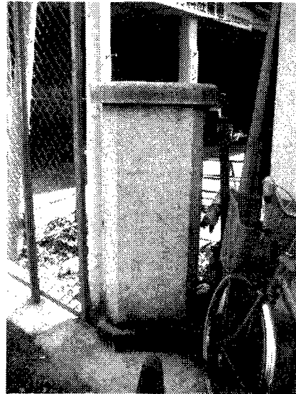
[写真-4.29：下流側右岸親柱]
