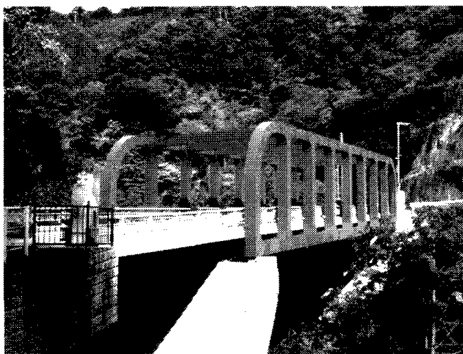
[写真-3.7.25：保津峡橋]
