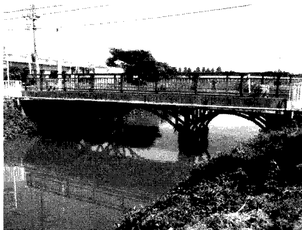
[写真-3.2.14：前屋敷橋]
